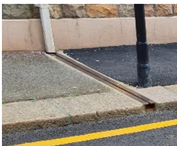
Metal water channel.
