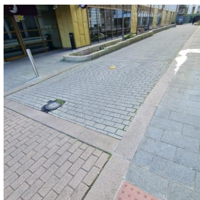
The carriageway and footway are defined by the row of kerb (Roxem different finish).
