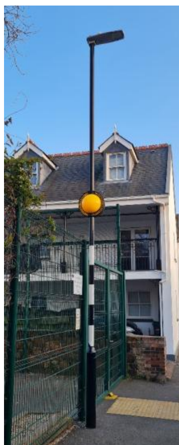
Example of Belisha beacon, which is integral with the street light fitting
