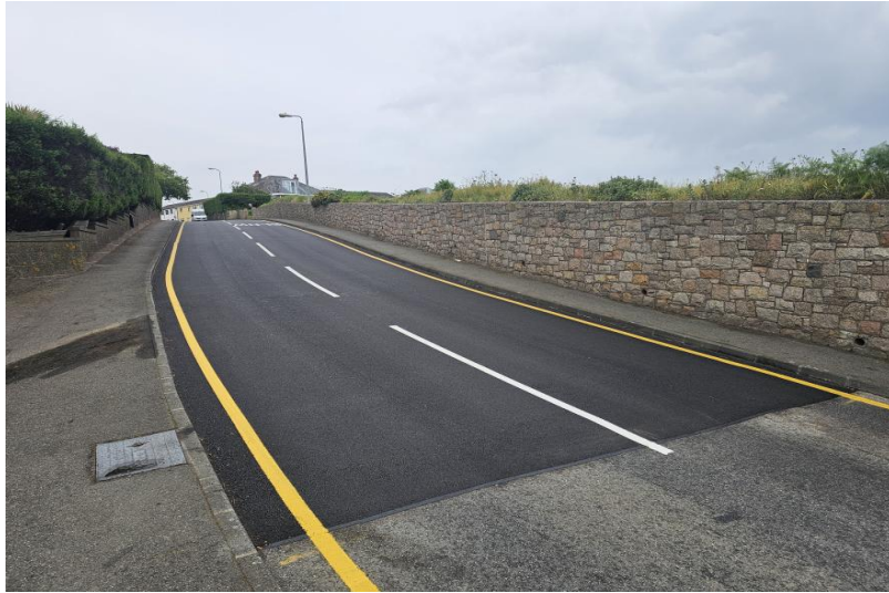
Tower Road - Panel of carriageway replaced
