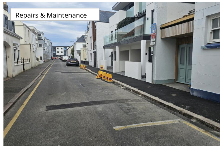
The department discussed with the developer to relay the footway as part of the redevelopment of the site - a lot of time spent by the department
