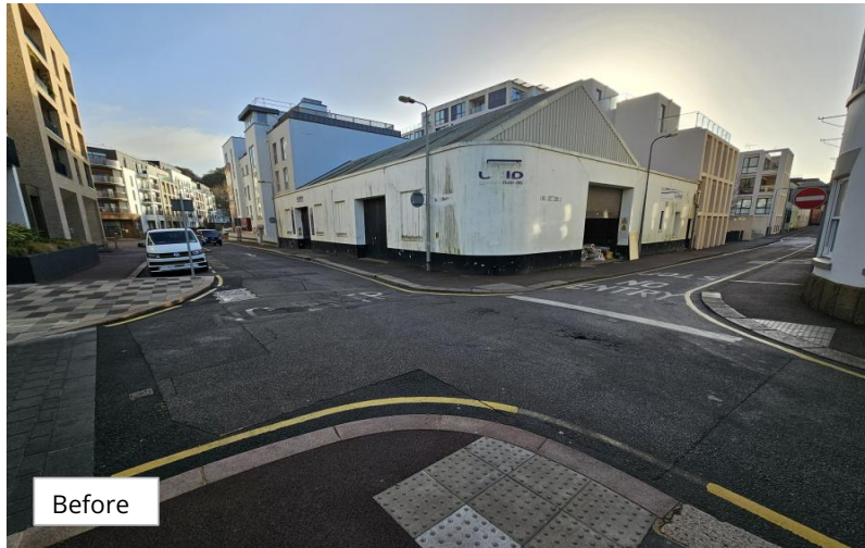
Charles Street - Large patch replaced to carriageway
