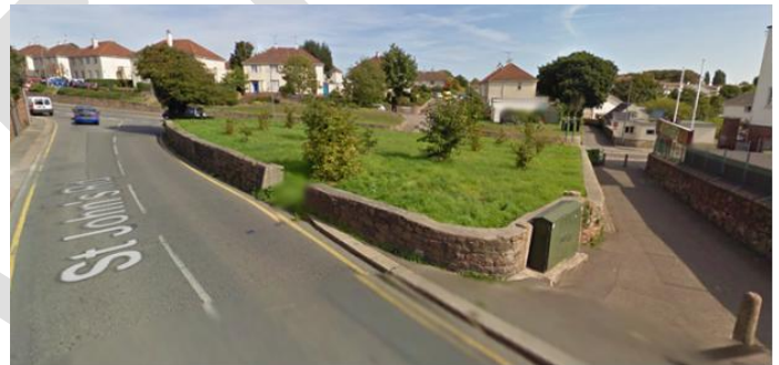
The existing La Chénée access forces pedestrians into the carriageway and has poor pedestrian visibility on exit.
