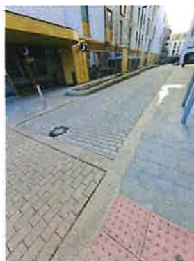
Roxem has been used for the carriageway in this private lane.
