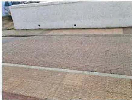
Roxem surface treatment used to indicate the speed humps/courtesy crossing.
