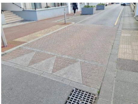
Roxem surface treatment used to indicate the speed humps/courtesy crossing.
