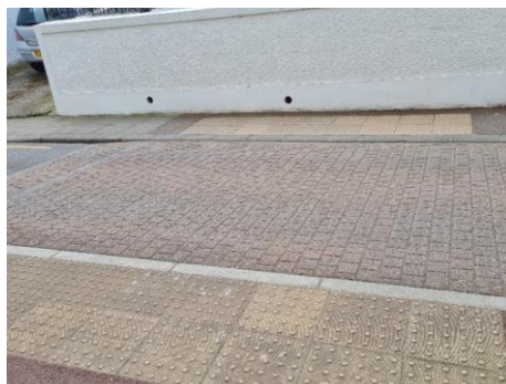
Roxem surface treatment used to indicate the speed humps/courtesy crossing.
