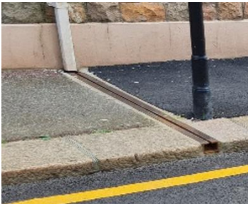
Metal water channel.
