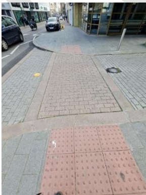
Used as a continuation of the footway, makes it clearer to pedestrians that they are approaching a vehicular entrance.
