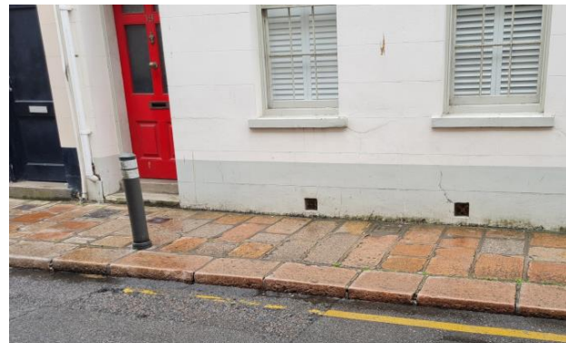
Example of the bollards placed in Don Street footway due to delivery vehicles mounting the footway. We propose the use of similar bollards in Lewis Street (south side)
