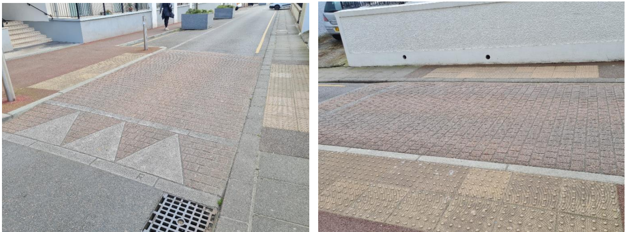
Roxem surface treatment used to indicate the speed humps/courtesy crossing.
