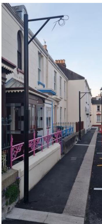
Example of hanging basket pole and arm, locally manufactured by 'JLS Fabrications'. The pole and arm were also powder-coated locally (Black). Irrigation system by 'Lawrence de Gruchy'
