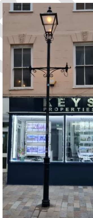
An example of the hanging basket arms being integral with the lamp column; however, in this example, the Parish had to use solar power lanterns as the irrigation pipe supplying water was run inside the pole, which could not be shared with an electric supply for obvious safety reasons.
