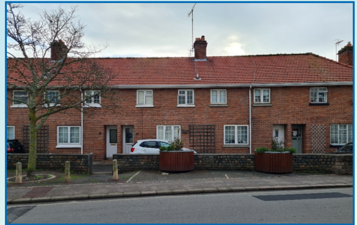
This photo shows the existing area unchanged, which will be the location of the proposed new exit.
