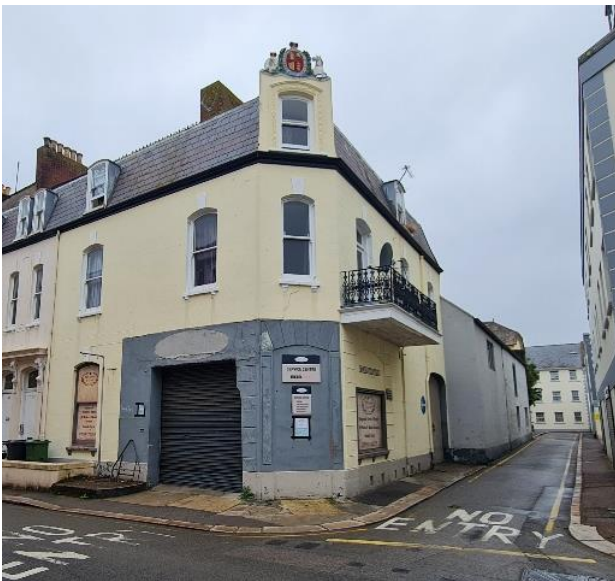
Photo of the former garage
