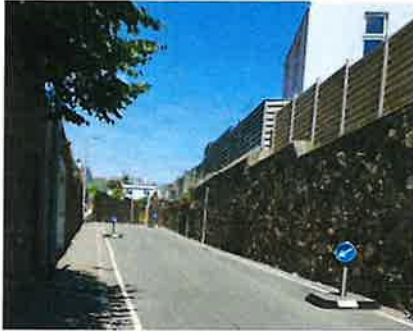
Before – chicane islands and narrow pavement
