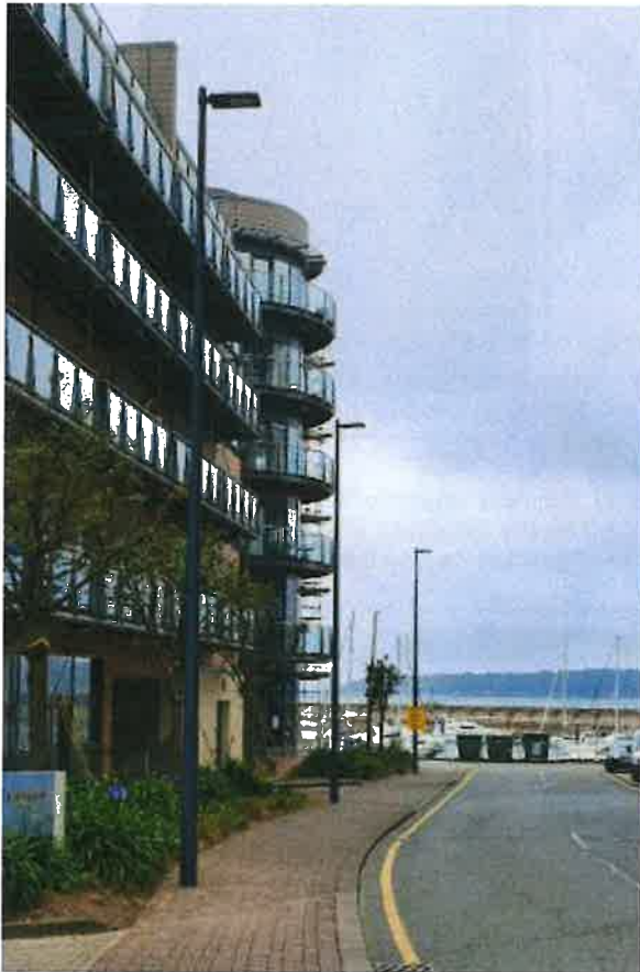
View along La Rue de Carteret showing consistent lighting scheme approach
