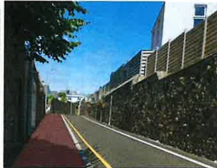
After – wider pavement for pedestrians, edge line moved away from wall opposite (artist's impression)
