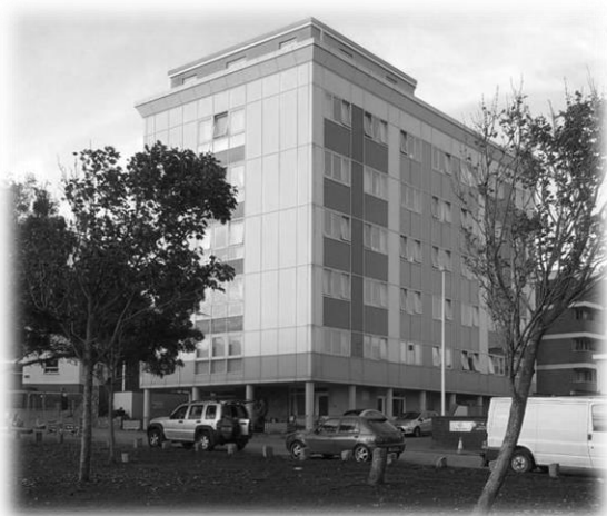
St Helier House
